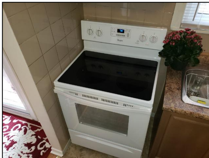
51. Anti-tip device missing
