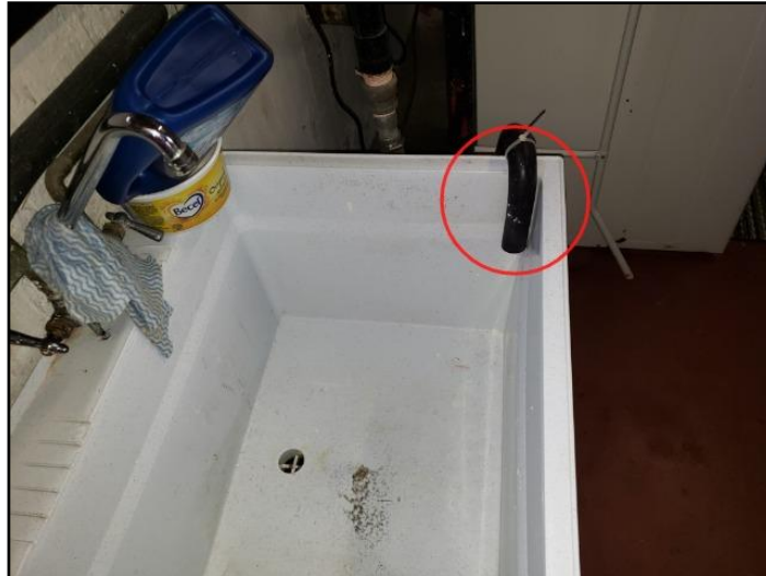
52. Standpipe missing
