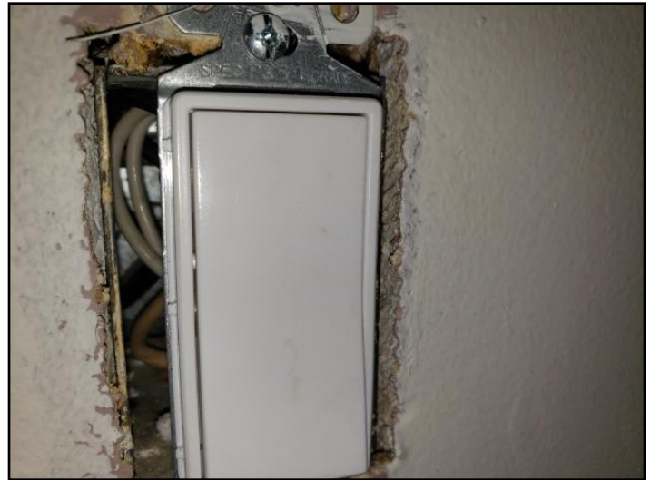
22. Connectors not compatible with aluminum
