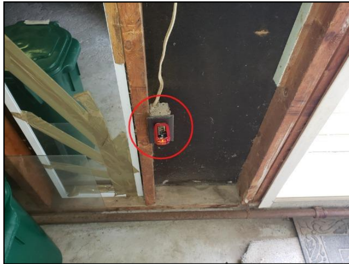
25. Reversed polarity
